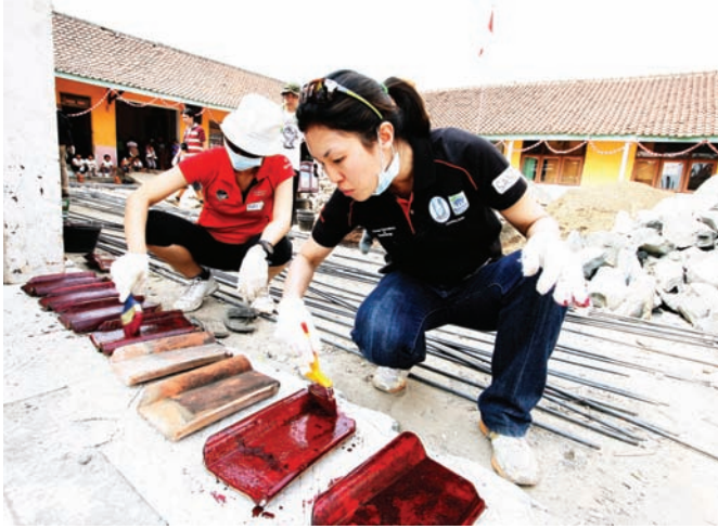
Our Group Operations and Technology colleagues painting the roof tiles of a classroom, part of a community development project to help build houses and a school at Banjaran, Bandung, Indonesia.
